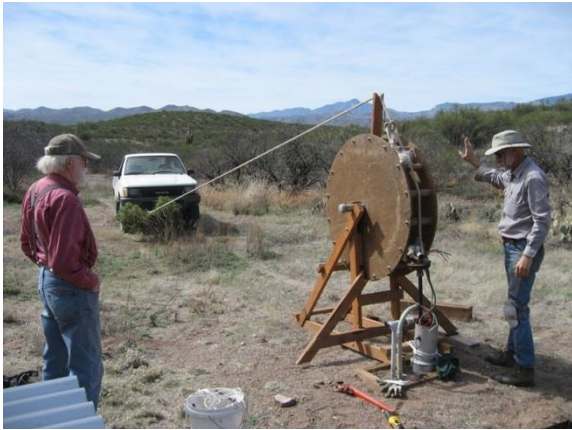
Pulling the pump from the well for repairs. David Omick, Gene Troutner & Pearl Mast driving.
